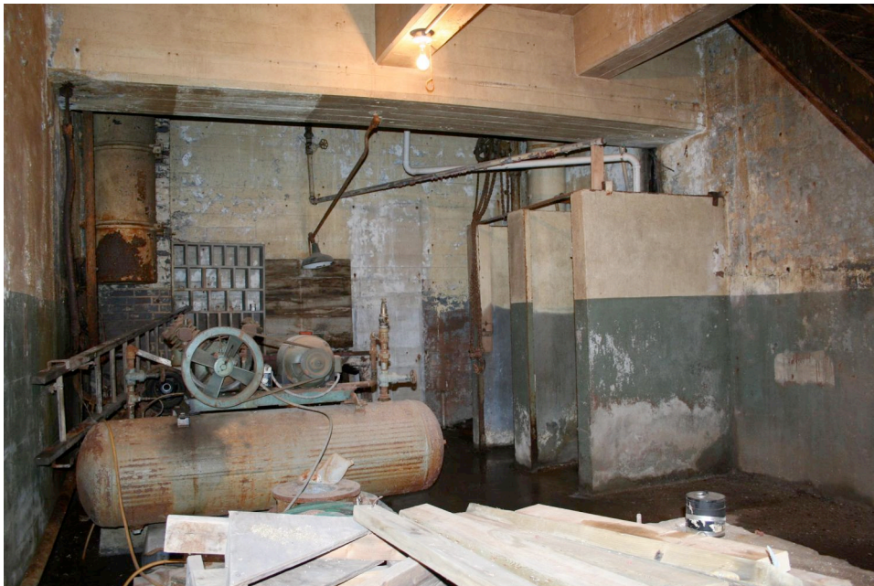
View of the lower level, looking south toward the showers and toilet stall used by the powerhouse personnel. Note the heavy concrete beams of the structural system.
