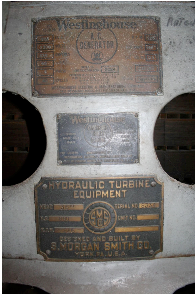
These identification plates located on the generators mark the equipment as designed and built by S. Morgan Smith Co., of York, Pennsylvania for the Westinghouse Company.
