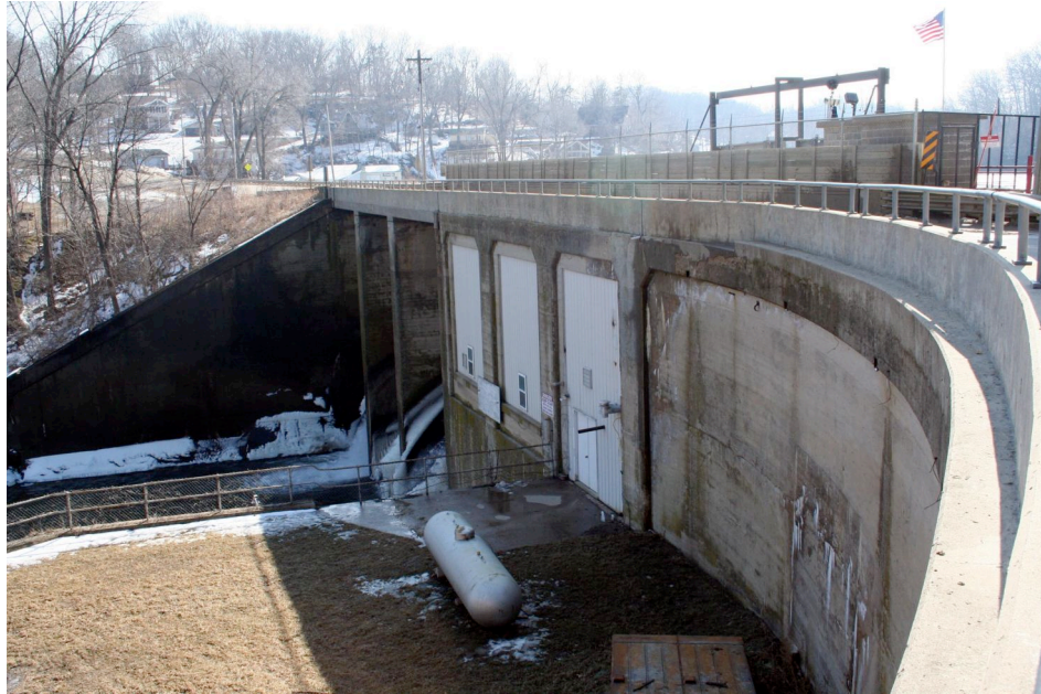
View of the downstream side of the dam and powerhouse, looking to the south. The concrete structure remains intact, with alterations made to the bridge's guard rail and the windows of the powerhouse - now filled with white, metal panels.
