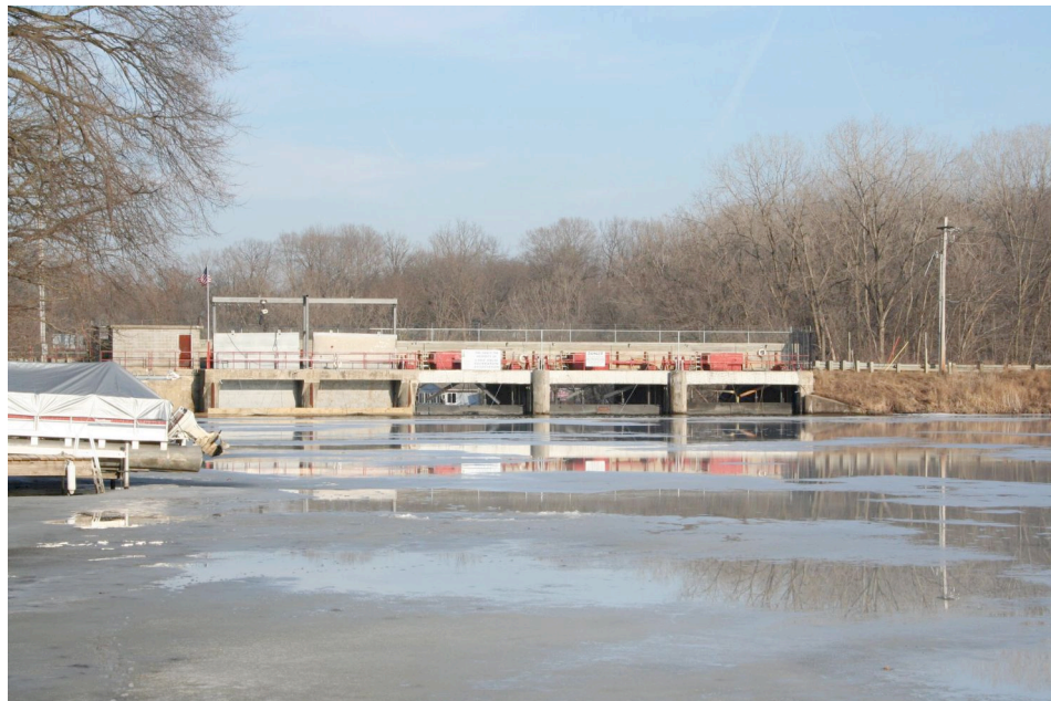
View of the upriver side of the dam, looking south from the lake. The three bays of the flood pass are located on the right and the two gates associated with the generation of hydroelectric power are on the left.
