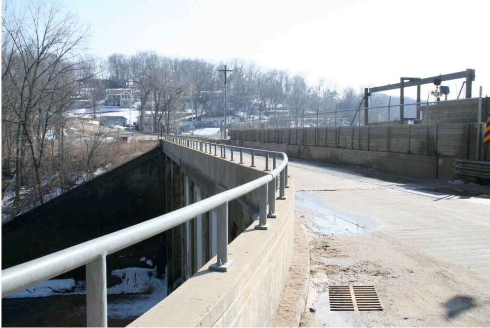
The dam and powerhouse are an integral part of the CR-X-31 bridge over the Maquoketa River. This view looks south along the bridge, with sections of the dam visible on either side.
